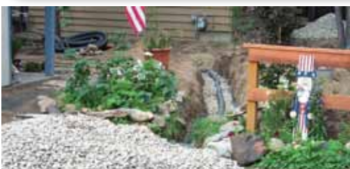
The area within 5 feet of your house is important to both water quality and defensible space concerns. When constructing erosion-control BMPs in this area, such as the installation of an infiltration trench shown at left, contact your local fire professional and Conservation District for advice on defensible space and BMPs.
